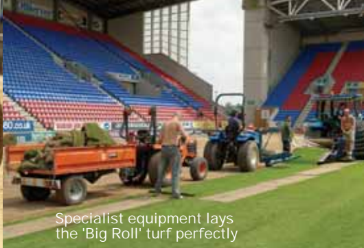
Like a huge jigsaw puzzle the turf interlocks for stability
