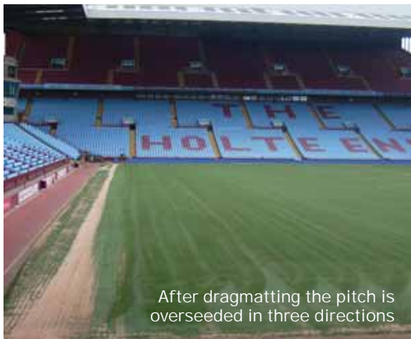
Sand is dragmatted into vertidrain holes
